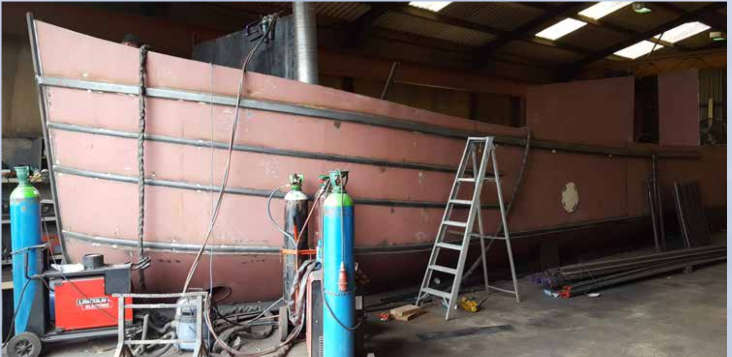
Steelwork for the hull almost complete
