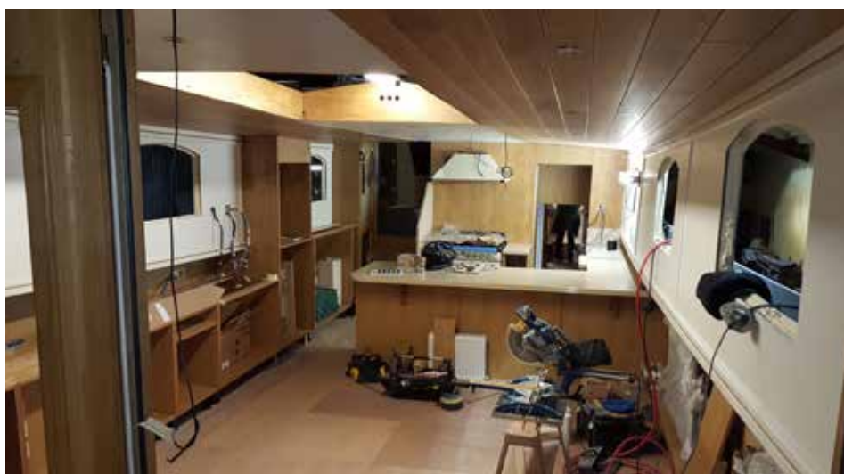
Interior spray foam insulation complete so fitting out gets under way
